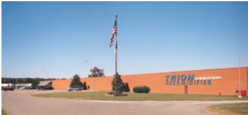
Corporate headquarters in Sanford, North Carolina
